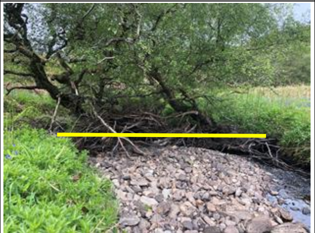
Fig. WGB1.6: View of the channel and both banks. The process of sediment aggradation is starting to develop naturally but more coarse and large woody structures are needed to connect the burn to the floodplain at much lower bank height
